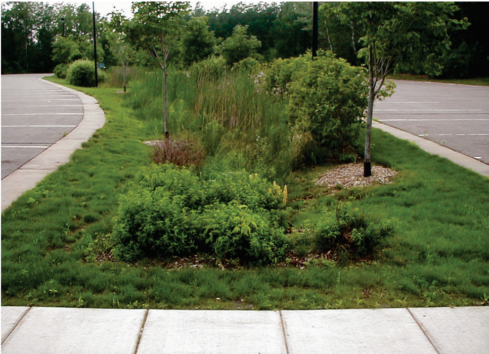
Parking Lot Bioswale
