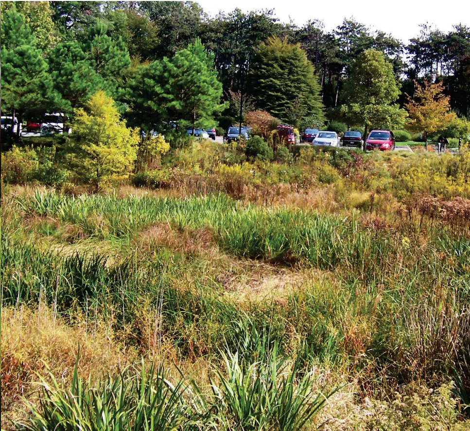
Dry (Detention) Pond
