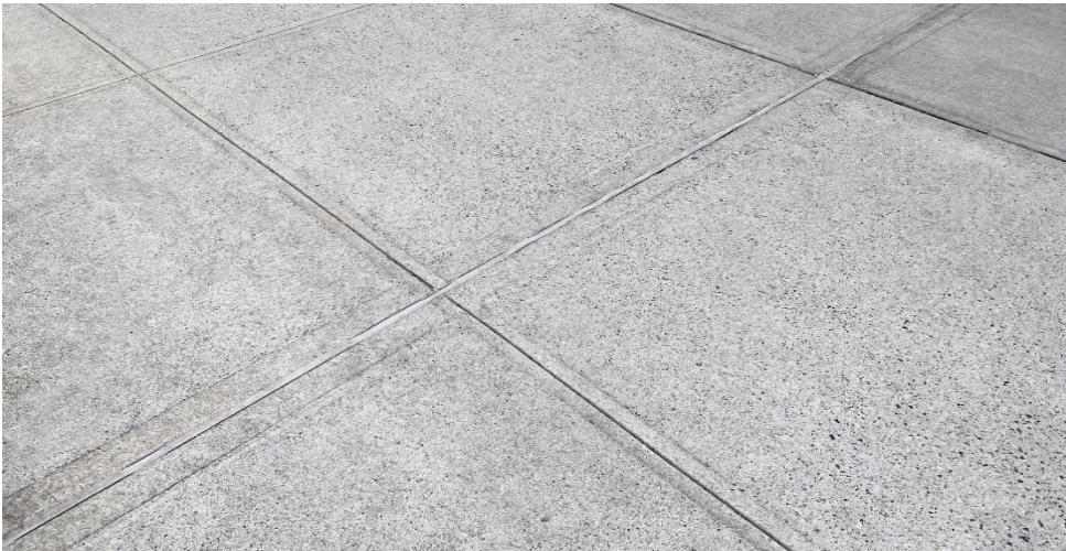
Regular cast-in-place concrete with broom finish and cut or tooled joints
