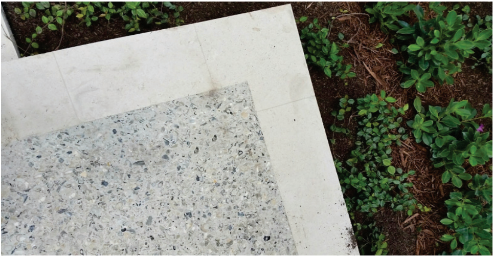
Cast-in-place concrete slab with integrated Tabby
