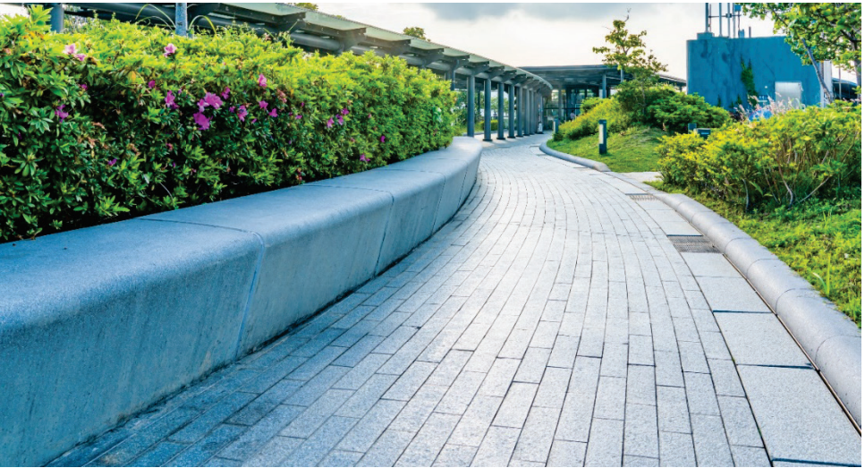
Precast architectural concrete wall
