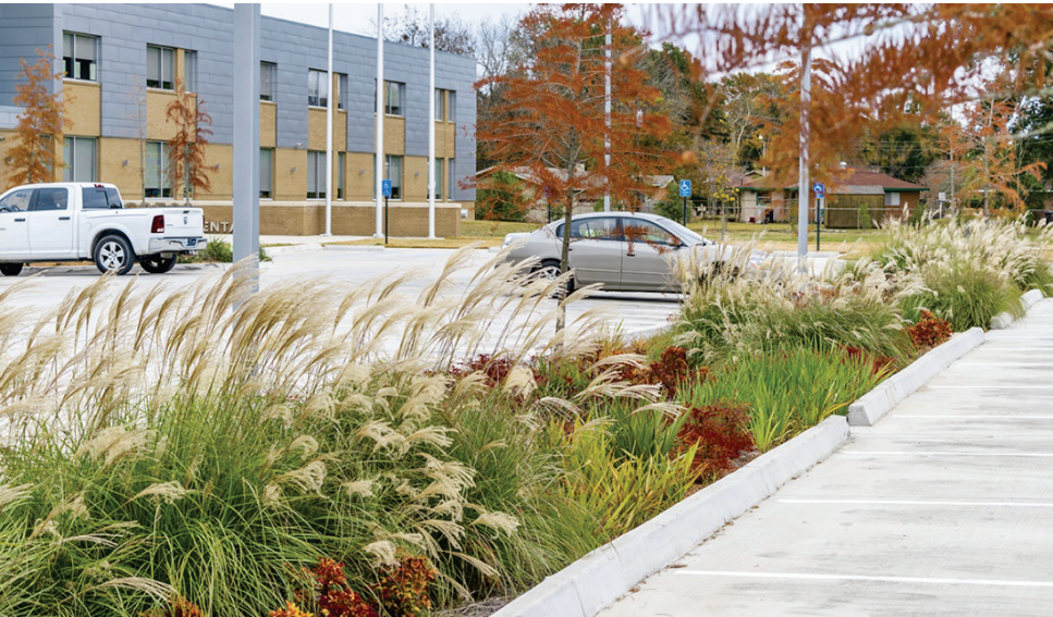
Native plantings in parking area islands
