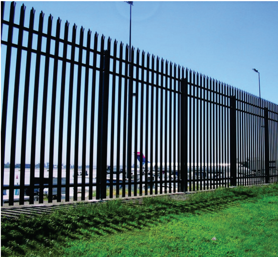
Type A – Powder-coated steel picket fence with a concrete mow strip. Use at Group 1 and 2 facilities.
