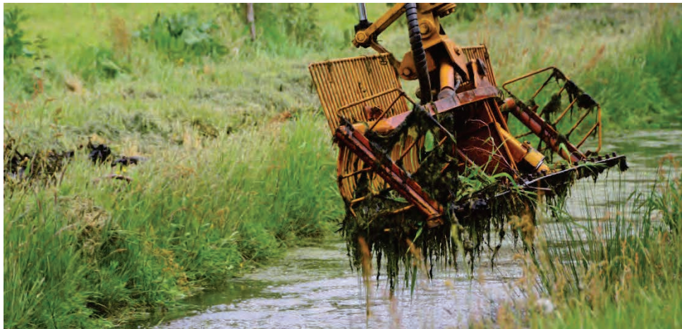
Removing silt and debris from channel
