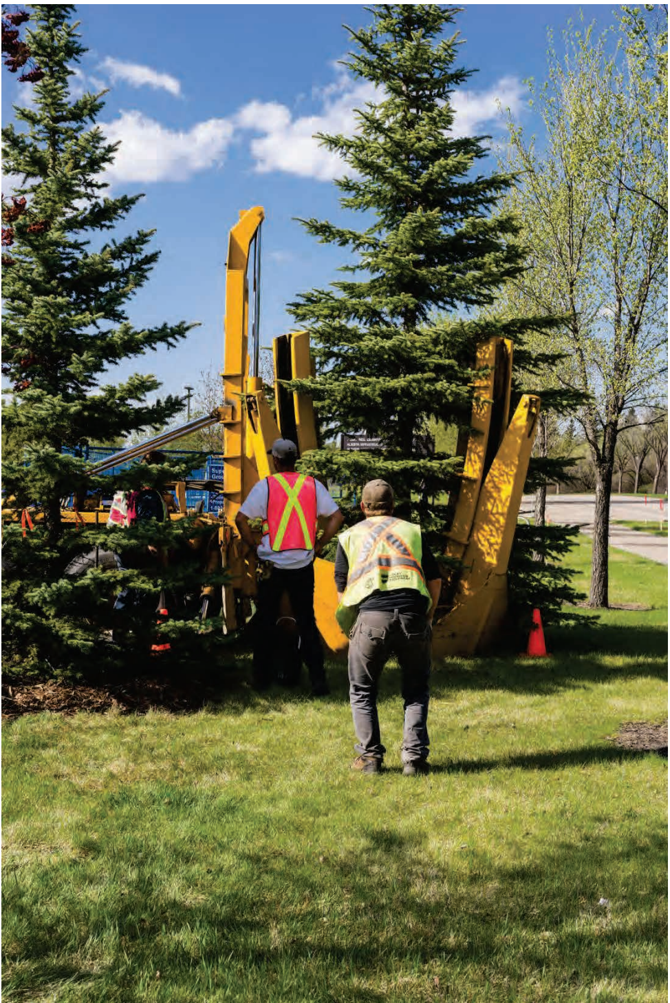
Transplanting trees will be done using a tree spade to prevent damaging the tree roots
