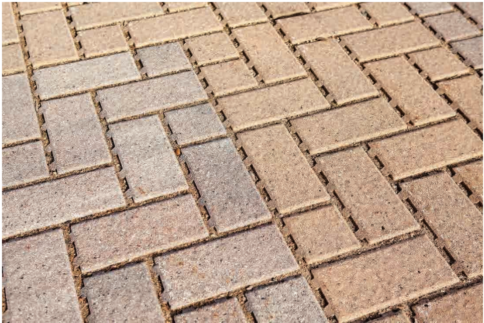
Clean joints between porous pavers and replace aggregate as necessary
