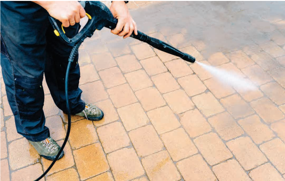
Set the pressure levels to be no greater than 500 pounds per square inch; perform two passes over surface of pavement, with wand spraying at a 45-degree angle
