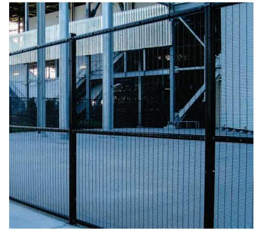
**Type C** – Powder-coated welded wire anti-climb security perimeter fence with a concrete mow strip.
