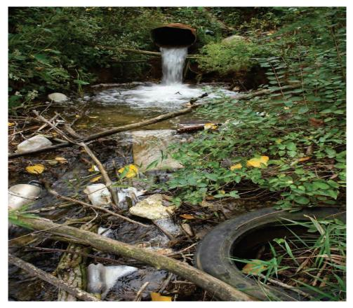
Remove all trash and debris from channel
