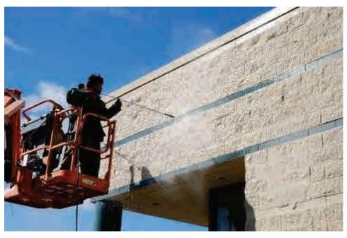
Use proper lift equipment to clean building face
