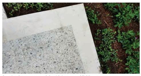
Cast-in-place concrete slab with integrated Tabby
