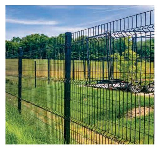
**Type B** – Powder-coated welded wire fabric security fence with a concrete mow strip. Use at Group 3 facilities.
