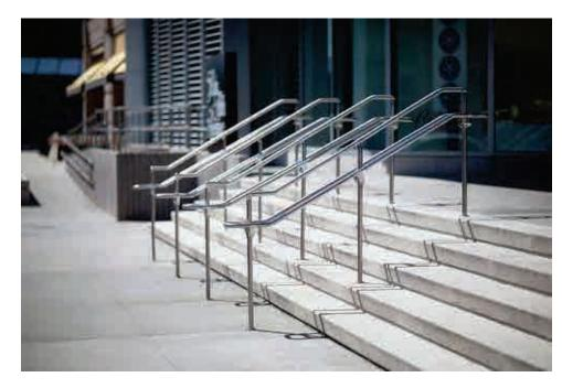
Cast-in-place concrete tread stair set
